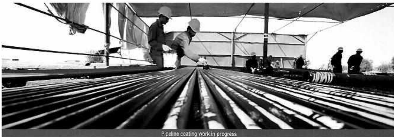
Pipeline coating work in progress
