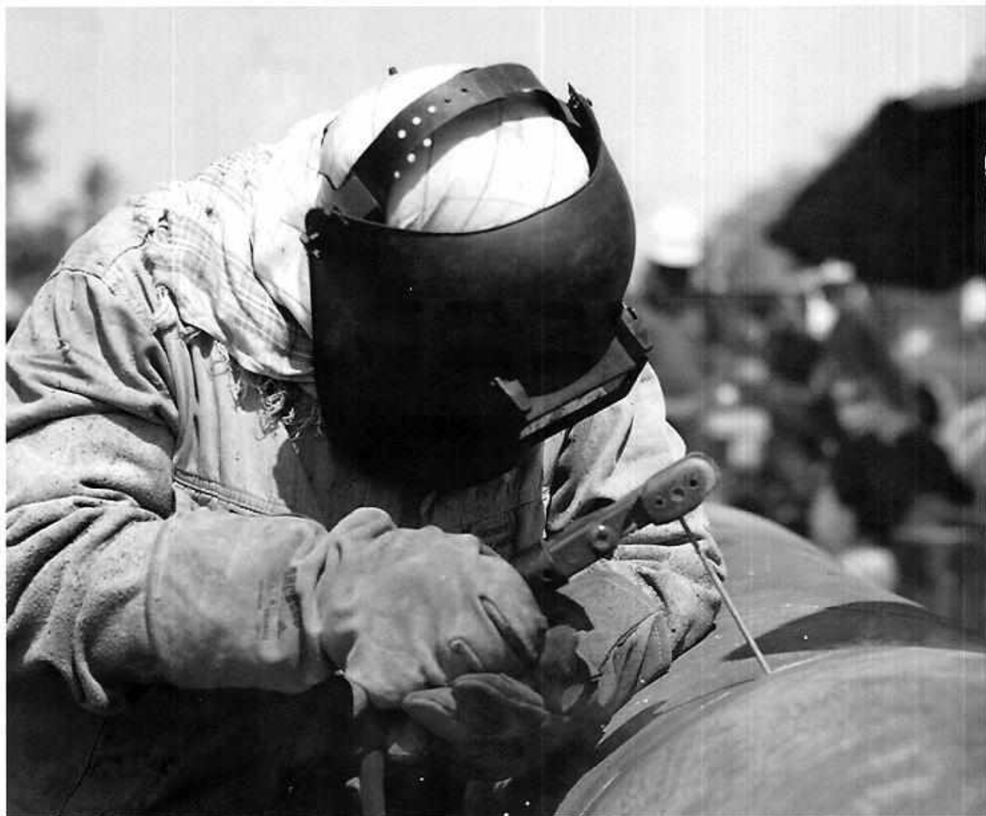
A tradition of commitment: A worker performing a joint weld during a pipeline laying in Balochistan in 1970
