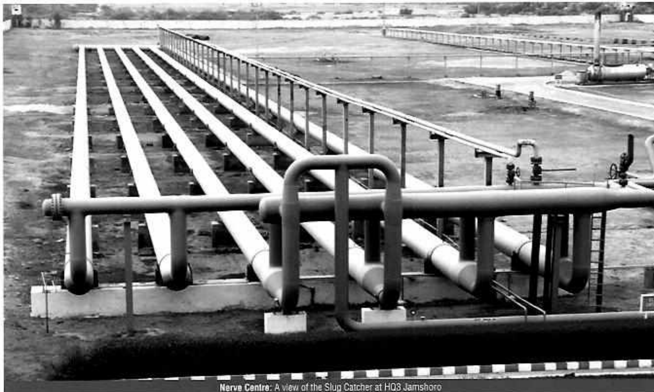
Nerve Centre: A view of the Slug Catcher at HQ3 Jamshoro
