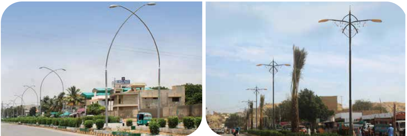
Streetlighting and plantation on the access road to Naya Nazimabad
