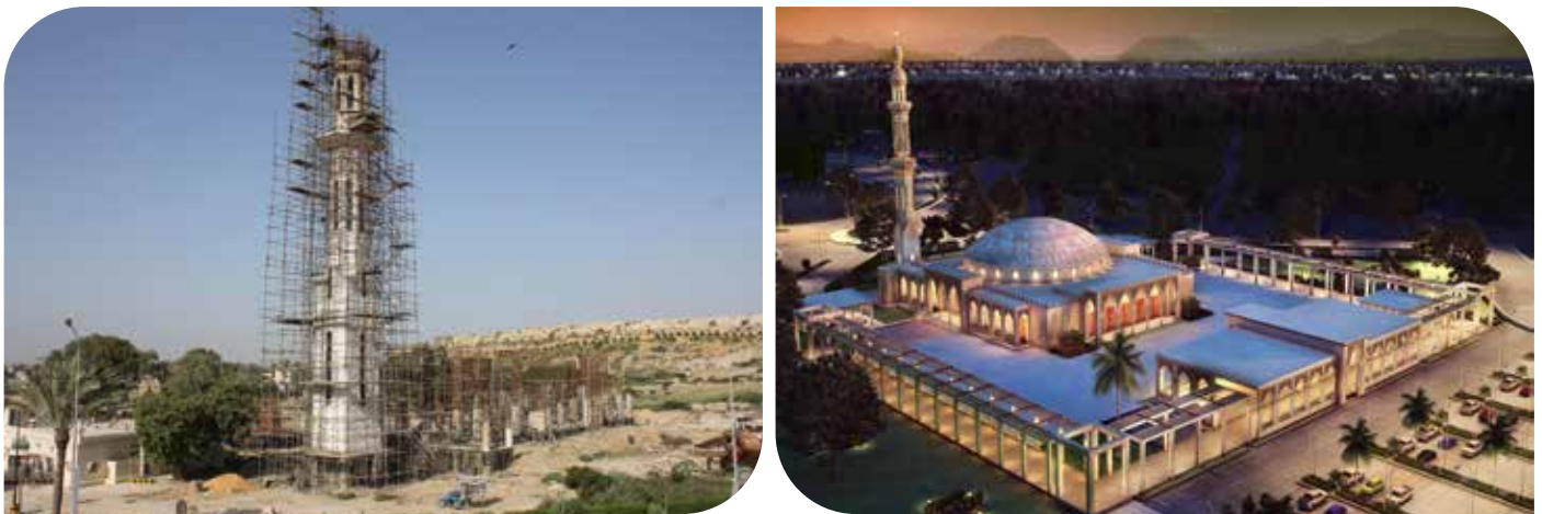
Construction of Central Jama Masjid
