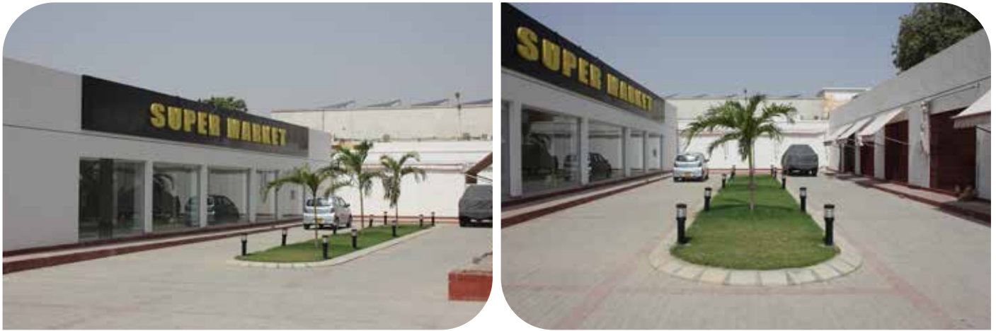
Completion of First Super Market adjacent to the Administration Block
