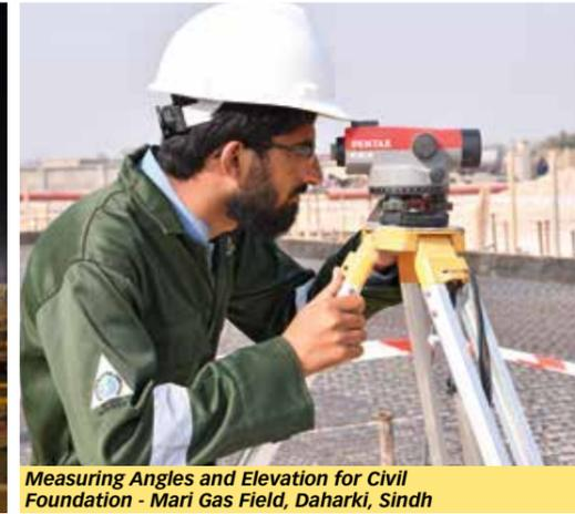
Measuring Angles and Elevation for Civil Foundation - Mari Gas Field, Daharki, Sindh
